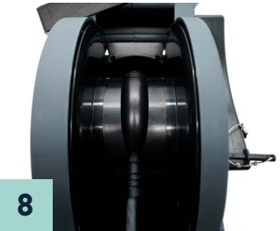
8 Final cable installation.
